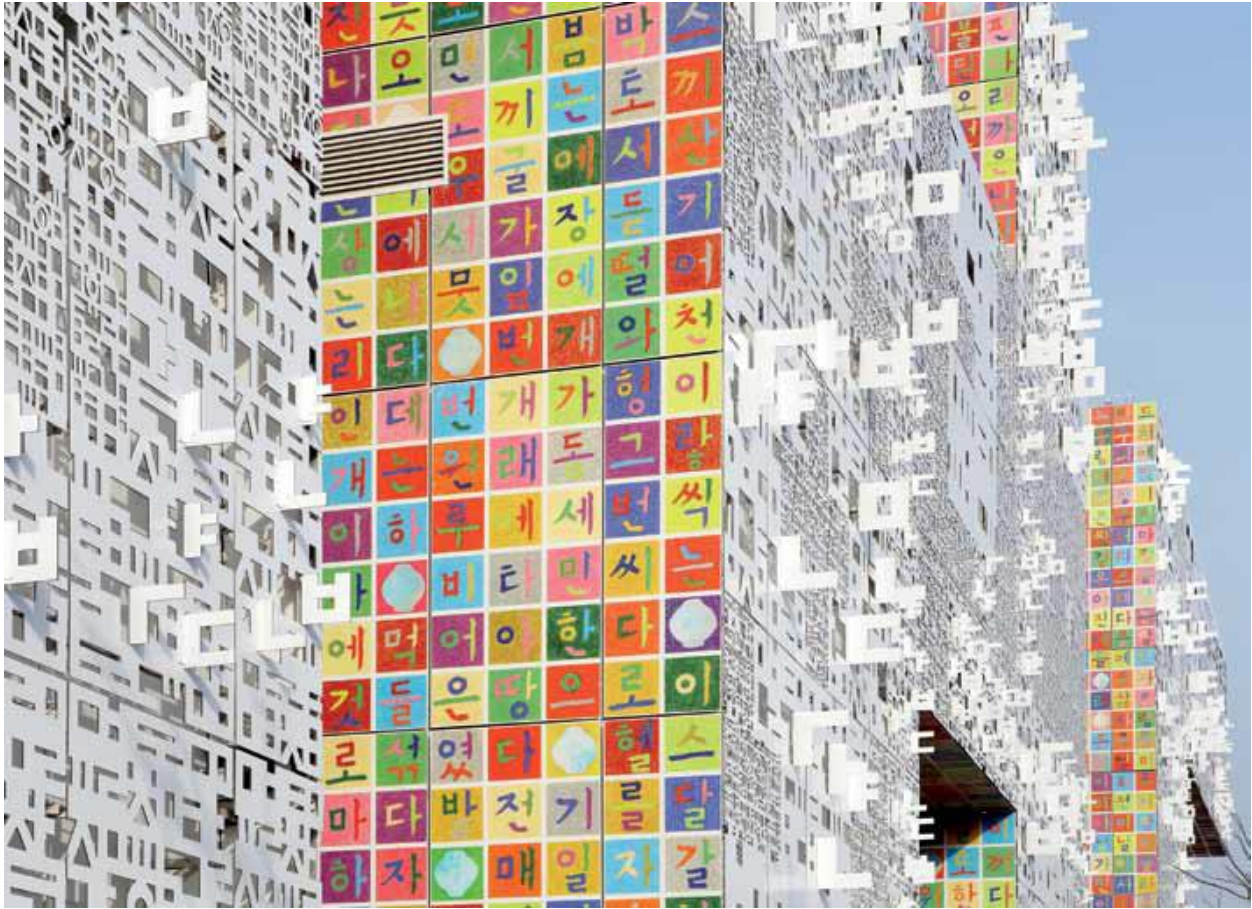
Mass Studies Korea Pavilion , Shanghai World Expo, 2010 Aluminum panels; computer numerical control
